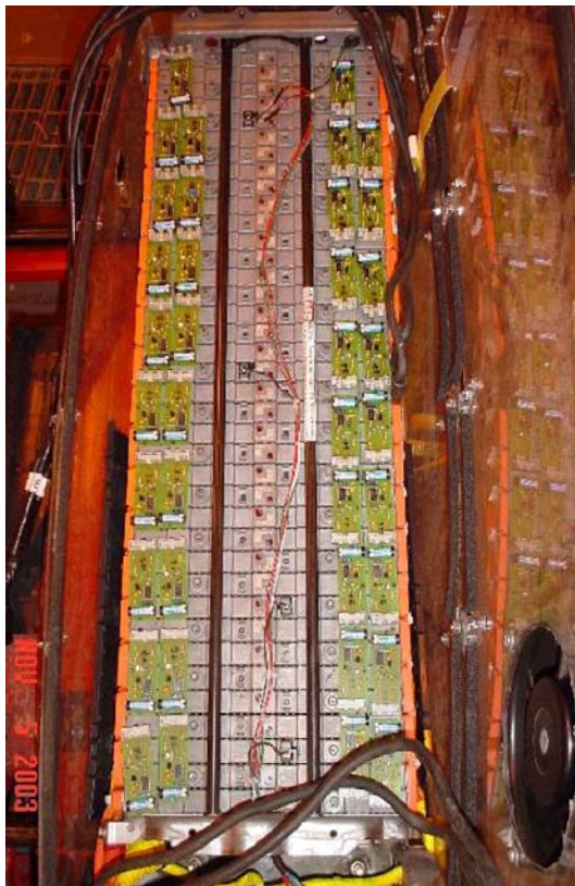
Figure 8. Battery Pack and Slave Boards.[15]
